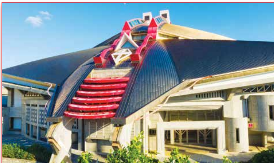
The Okinawa Prefectural Budokan is located on Hwy. 58 within easy walking distance of Asahibashi, Tsubogawa, and Onoyama Koen monorail stations. The CFA/Rengokai seminars will be held there until construction of the World Headquarters of Karate ( Karate Do Kaikan ) in Okinawa is completed.
